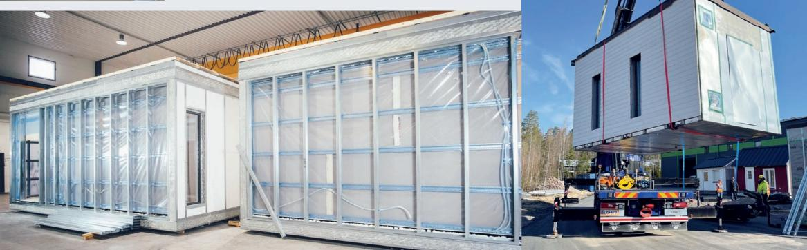
All modules are assembled indoors in Aulis Lundell's production facilities and are ready to use after placing on the foundation and connected to utilities. All steel components are fabricated according to high-quality standards and accurate dimensions, and all elements and modules have precise small tolerance dimensions. Joining modules together is easy and requires no adjustment work at the site.
